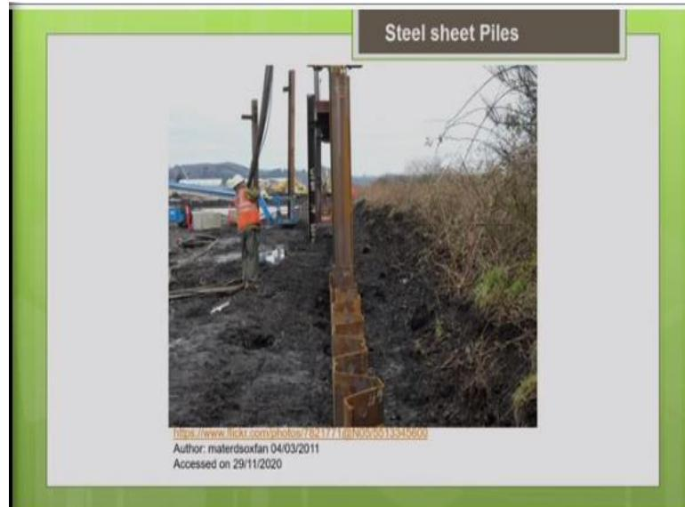
So, this is again a picture of the steel sheet pile, you can see the interlocking joints. So, this is mostly driven with the vibrating hammer, what is this vibrating hammer all these things? We will be discussing in the part 2 of this lecture, so where we will be discussing about different types of pile hammer. So, this helps to support a lateral load from the soil, helps as a barrier to the earth.
